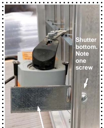
Shutter Motor Bracket (bottom view)
